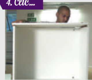
Top panel into place
